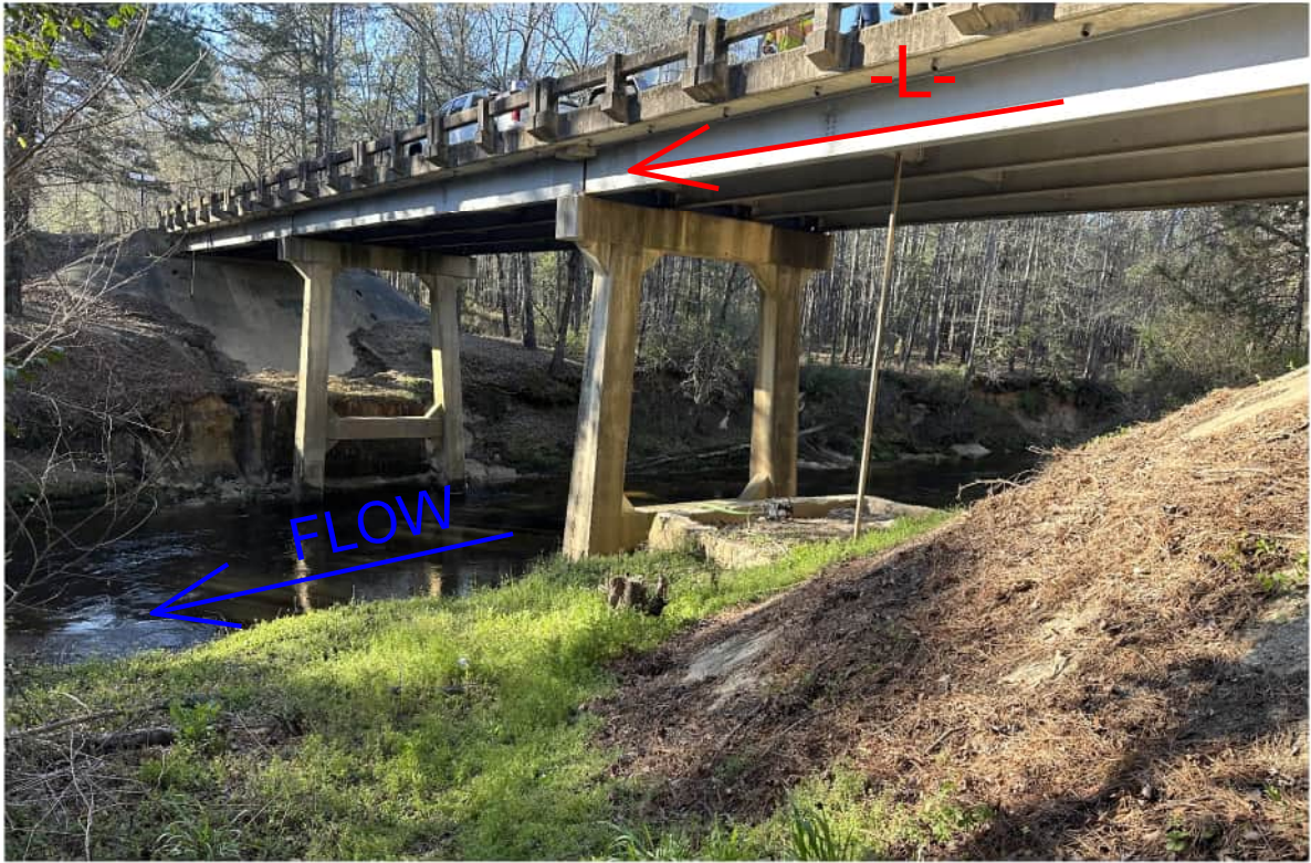
NORTH SIDE OF BRIDGE LOOKING SOUTH (UPSTREAM)
