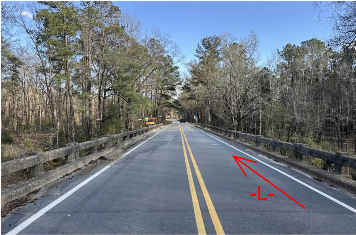
WEST APPROACH LOOKING EAST ALONG -L- ALIGNMENT
