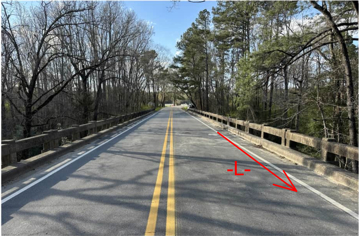
EAST APPROACH LOOKING WEST ALONG -L- ALIGNMENT
